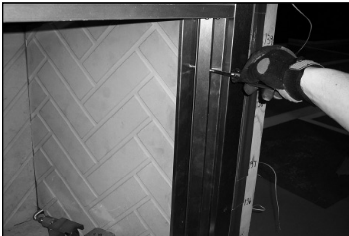
Figure 6.3 Loosen Refractory Retaining Strip
